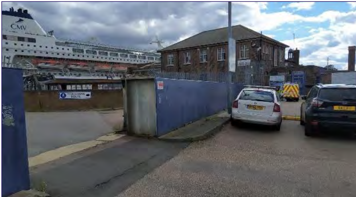
Figure 6-3: London Resort Essex Project Site existing flood defences (photograph taken during site visit 28/07/20, looking west)
