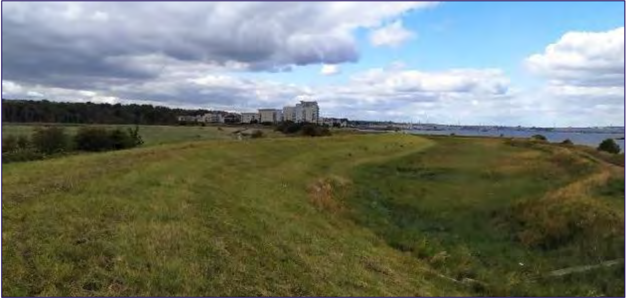
Figure 4-3: Kent Project Site (Main Resort) existing formal flood defences at Black Duck Marsh (photograph taken during site visit 28/07/20, looking southwest). Black Duck Marsh to the left side of photograph and the old flood defence embankment alignment on the right side.
